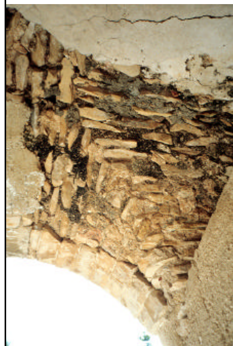
Liaison Ossature – Structure Verticale
